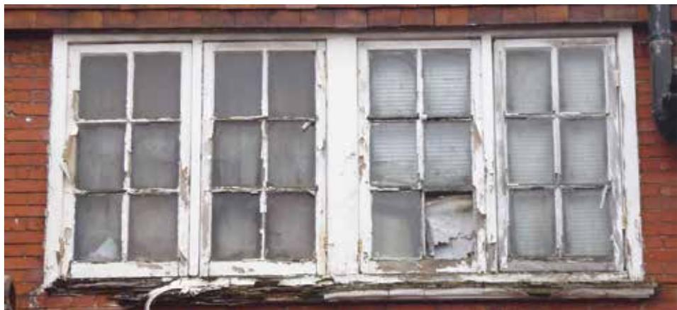
Above and right: Examples of severely deteriorated casement windows. These windows could be replaced under the LLBCO.
