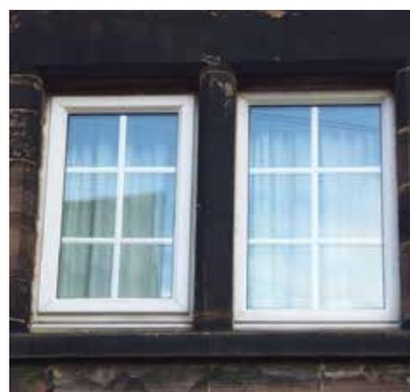
uPVC windows are inappropriate and were installed without consent. To address this enforcement issue, these windows could be replaced under the LLBCO.
