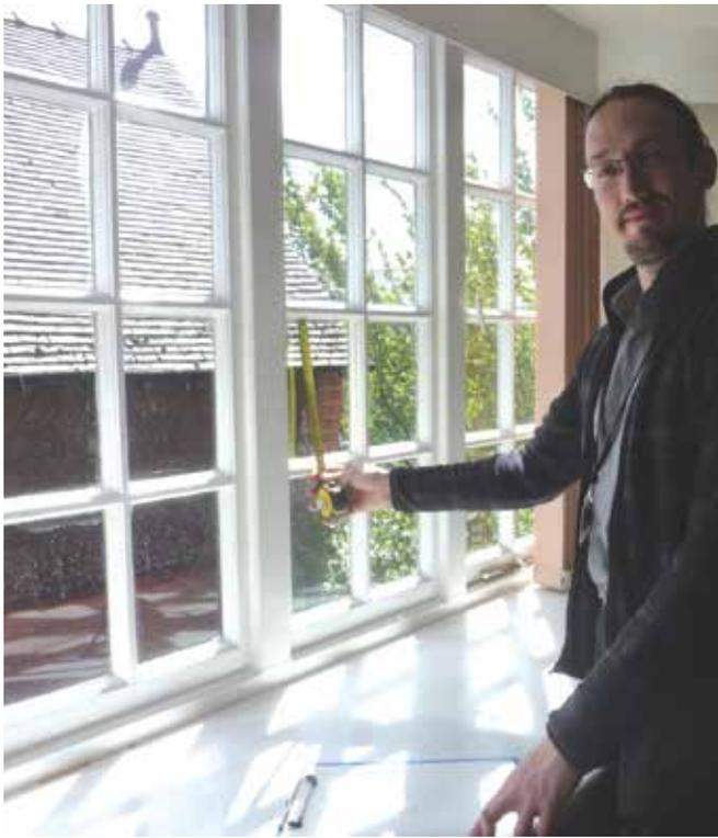
Paul Hetherington, Architectural Technologist and Building Surveyor, Wirral Council, is shown measuring the 8 light casement windows at 95 Greendale Road. Paul used the measurements to make the drawings shown below. Your drawings need not be computer generated. Hand drawn sketches are fine as long as they are clear, to scale, and show key dimensions.
