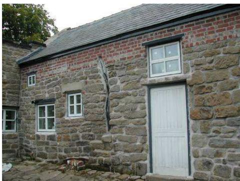
*Barn to Stone Farm; stone with cruck frame evidence. Brickwork possibly resulting from lowering the roof pitch following replacement of thatch by slate.*
