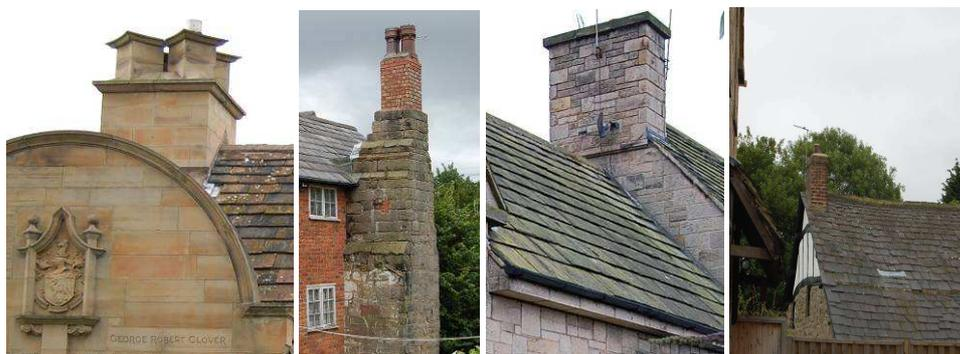
*Chimneys in the conservation area; (1) Clover Cottages (2) stone with sections rebuilt in brick seen extensively (3) simple copings to stone chimneys(4) plain brick stack.*
