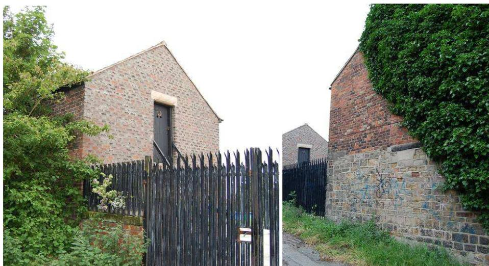
*(left and right) poor quality pointing to stone and brickwork as well as highly detrimental palisade fencing at Ivy Farm.*
