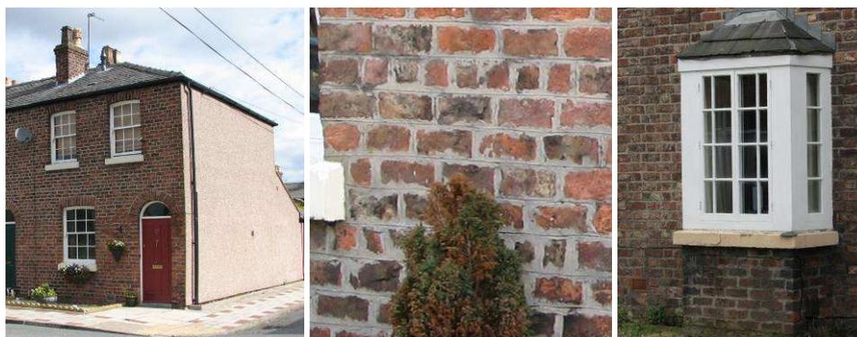
*Unsympathetic alterations within the conservation area: (left) pebbledashed end walls to the terraces; (middle) poor quality pointing; (right) the effect of installing double glazing – making the window frames wider, therefore leading to an odd configuration of glazing bars.*
