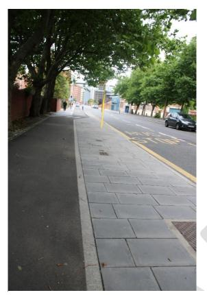
Picture 3.2 Separated cycleway with floating bus stop, Park Lane, Liverpool
