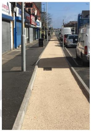
Picture 3.3 Separated cycleway with floating parking bays, Duke Street, Wirral
