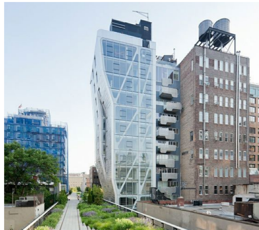
Figure 6.4.5 - Landscape framing views - Highline New York - Field Operations
