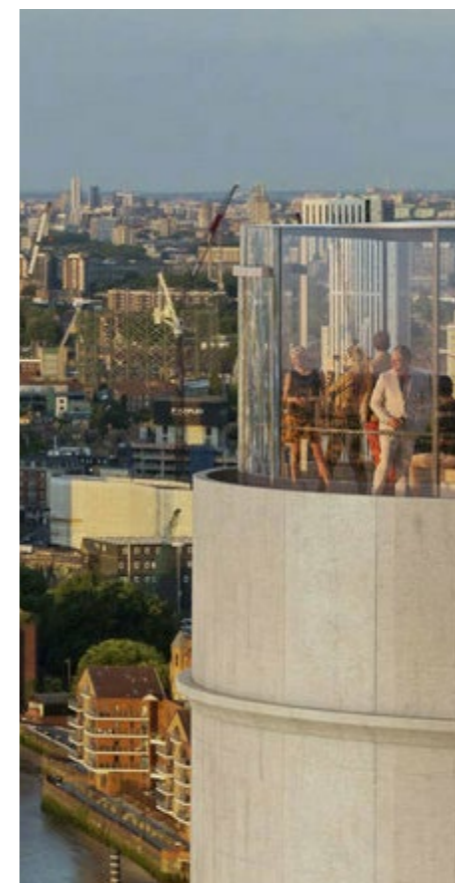
Figure 6.1.10 - Battersea Power Station Lift
