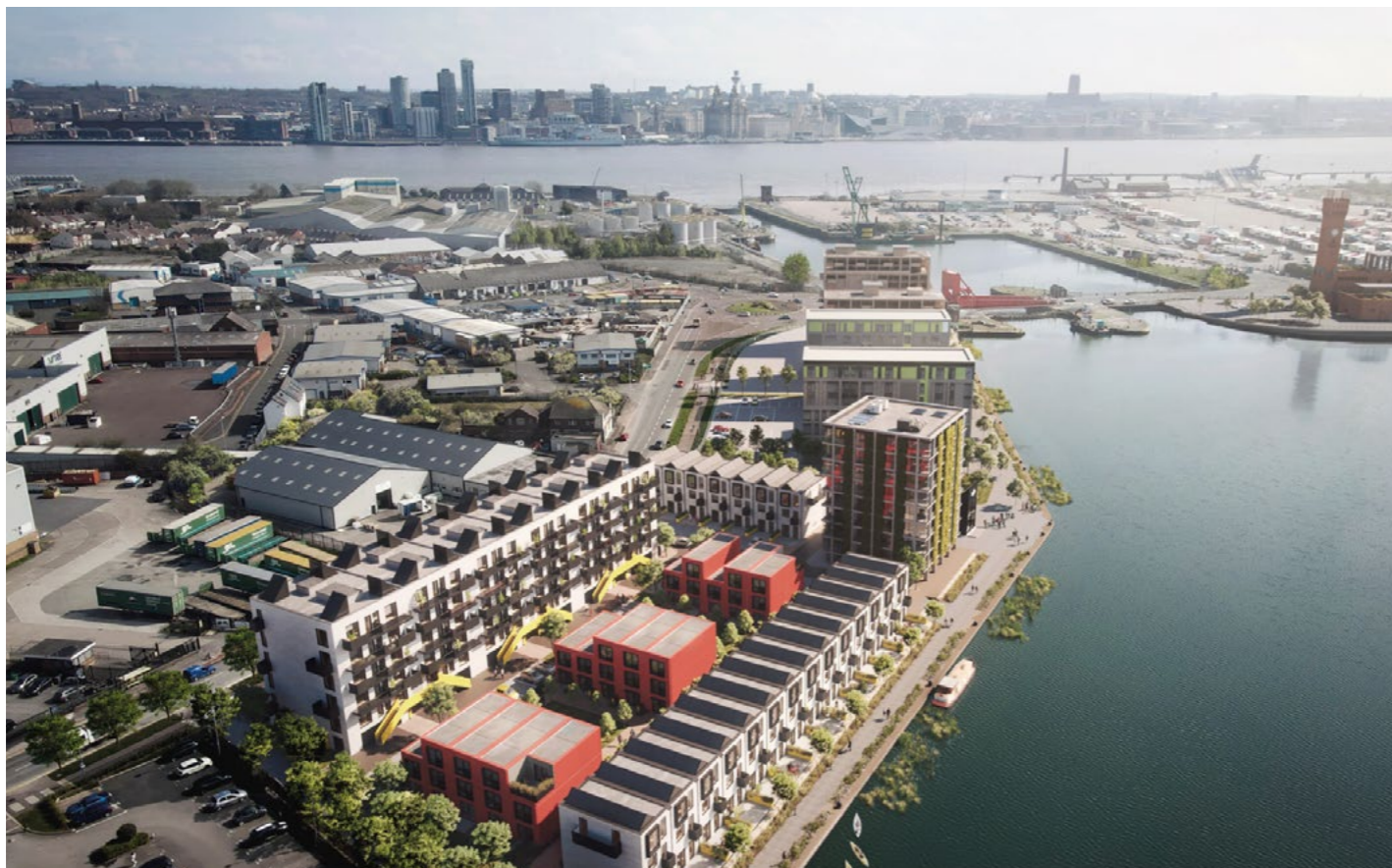
Figure 5.12.3 - Redbridge Quay in Wirral Waters
