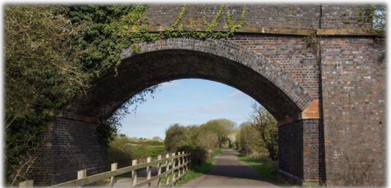
Dungeon Bridge on the Wirral Way, looking towards Thurstaston
