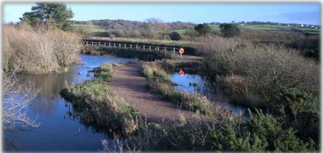
Part of a Natural England funded project in 2022 was to install a fully accessible path through the nature ponds within the Dee Cliffs Site of Special Scientific Interest
