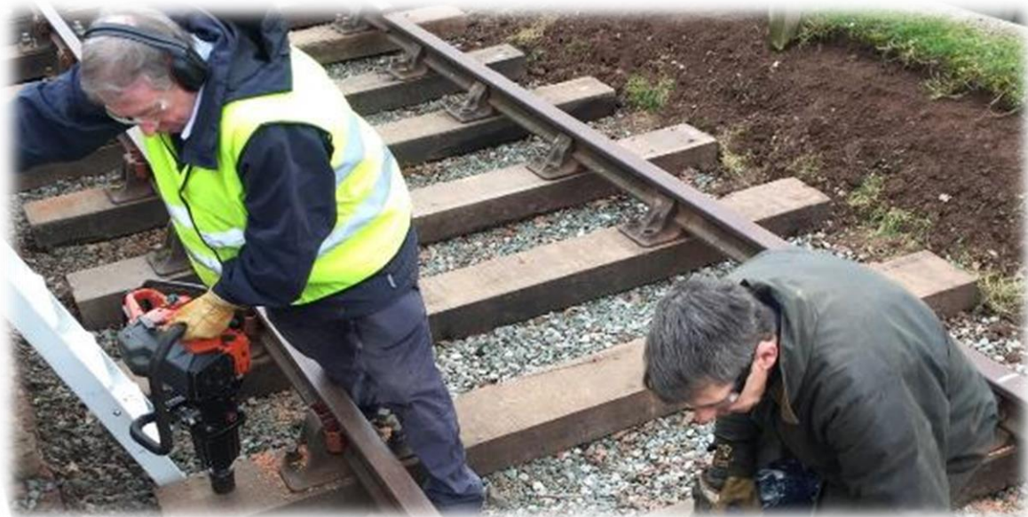
The friends group installing new sleepers along the restored trackbed
