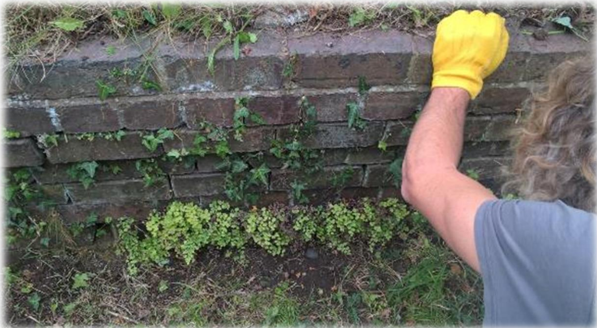
Re-pointing of brickwork requires careful management alongside species recorded as part of the Local Wildlife Site (Site of Biological Importance)
