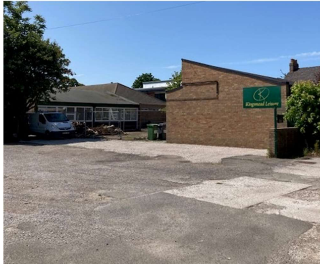
Site visit June 2025 - buildings and car park
