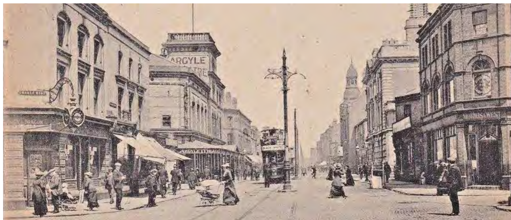
Argyle Theatre and Grange Road
