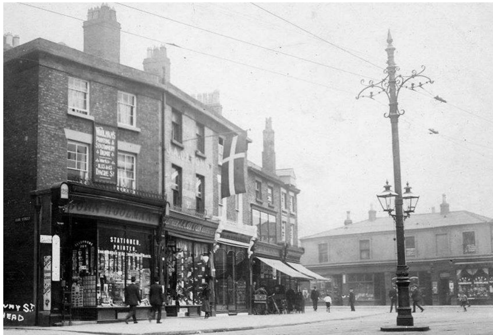
Conway Street and Argyle Street Junction
