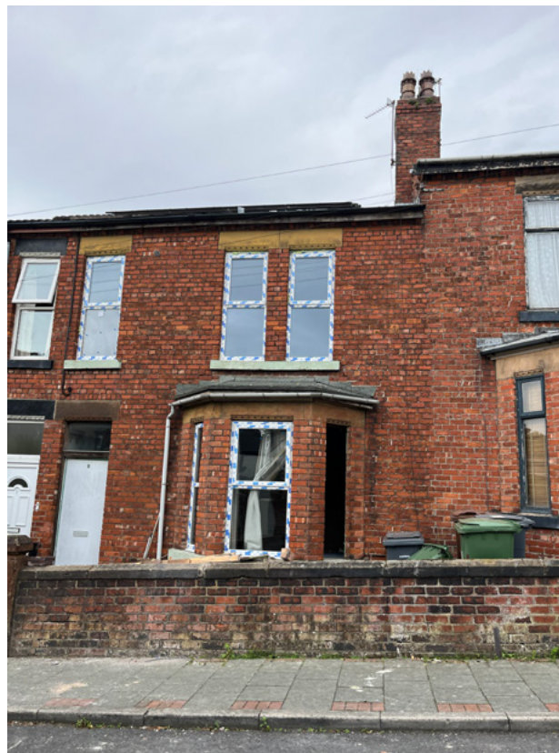
4.3.44 Simple stone dressings with later UPVC windows to terracing
