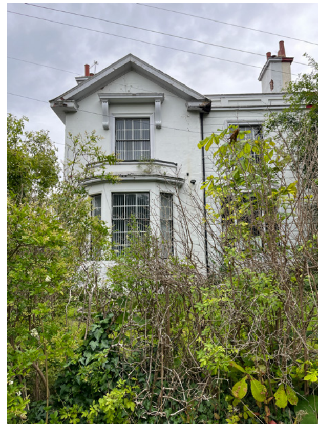
4.2.16 Heavy classical eaves
