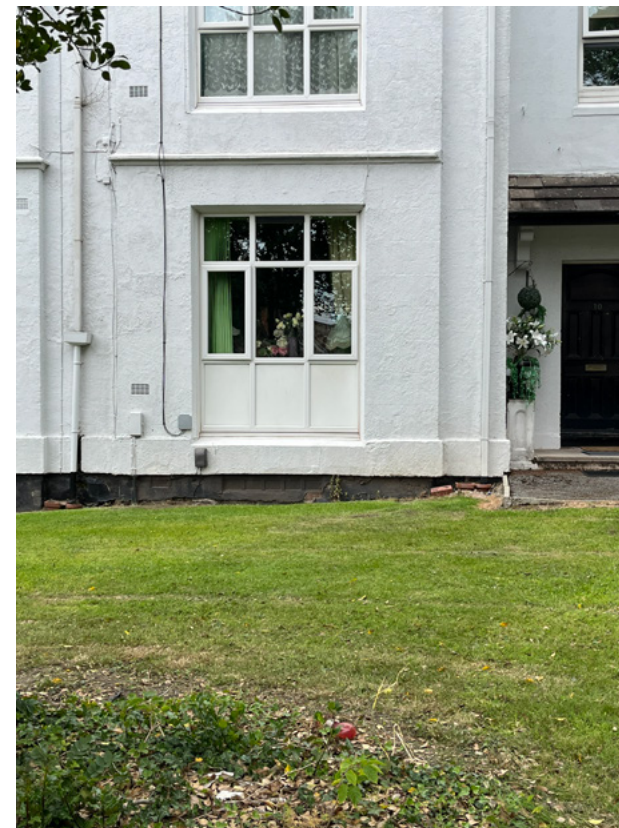
4.2.10 UPVC windows in historic bay
