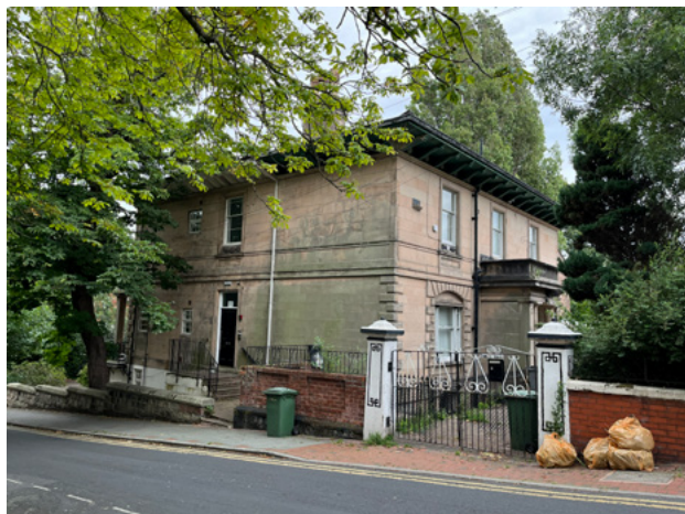
4.3.4 Rear of 47-49 Clifton Road
