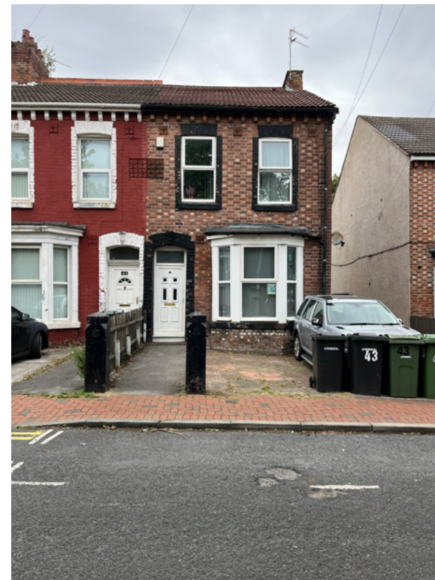
4.3.28 19 th century typical terrace
