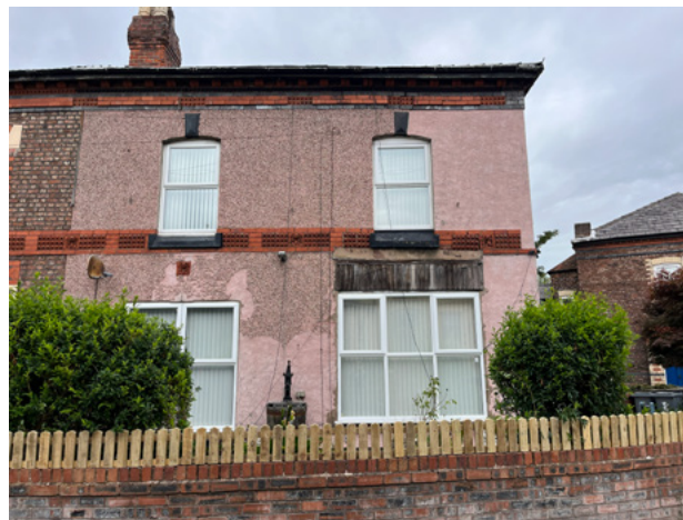
6.3.2 Some houses have been covered with render
