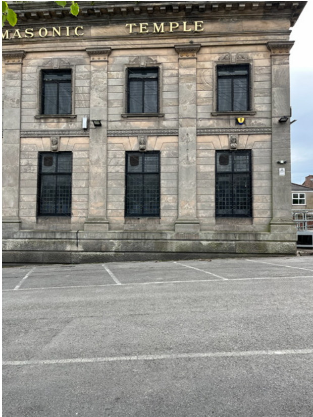
4.3.18 Large pilasters to former Masonic Temple
