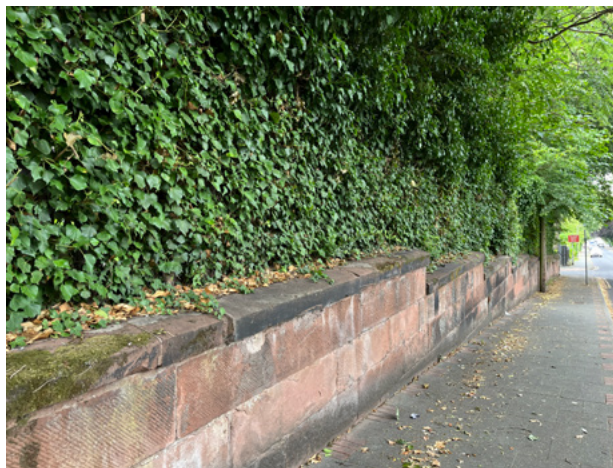
4.2.23 Sandstone boundary to Clifton Road
