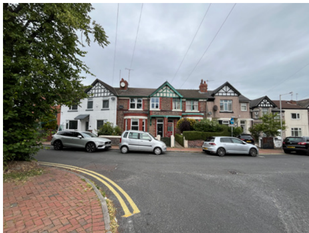
4.3.29 Typical block of late 19 th century terracing
