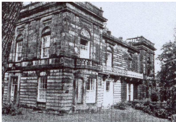
3.1.12 38 & 40 Clifton Road prior to demolition, 1982 (DIA)
