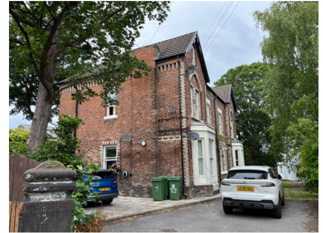
4.3.40 Typical building to Circular Road
