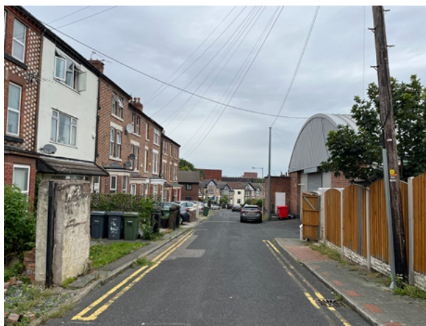
4.3.49 Poor quality public realm and Drill Hall to right
