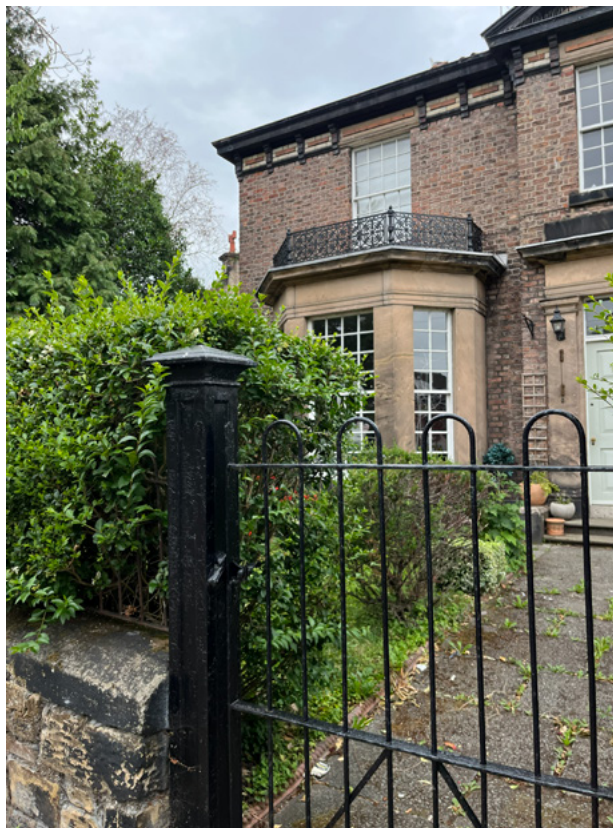
4.2.9 Historic canted bay
