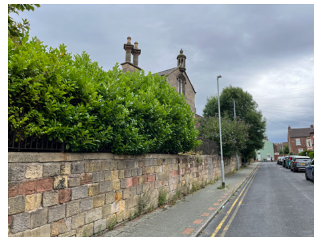
4.3.50 View of boundary wall and apex of Fearnley Hall gables
