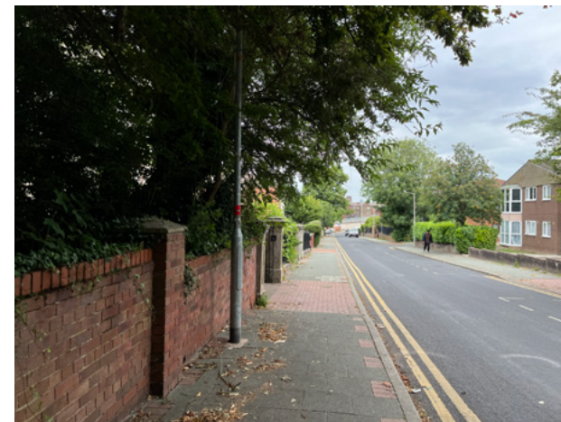
4.2.19 Blockwork paving to Clifton Road
