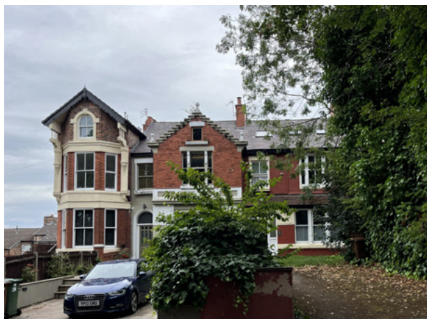
4.2.8 Vernacular revival house to Clifton Road
