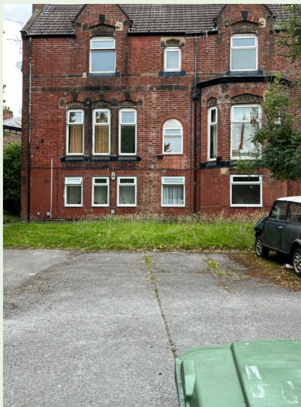
6.2.2 Modern UPVC replacement windows
