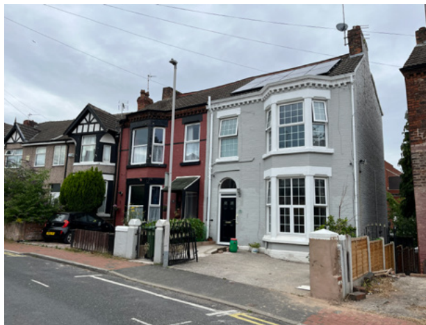
4.3.30 Contemporary paint to brickwork of late 19 th century terrace
