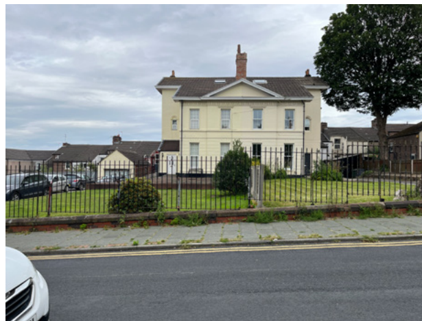
5.3.7 Views of between buildings to rear of Rodney Street
