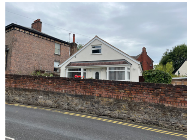
4.3.45 Mixed brick and rubble masonry wall to bungalow
