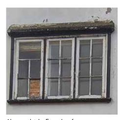
Above and right: Examples of severely deteriorated casement windows. These windows could be replaced under the LLBCO.
