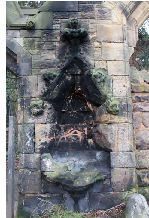
There is evidence of the water fountain on the external wall of the gate. Note the vandalism and fire damage.
