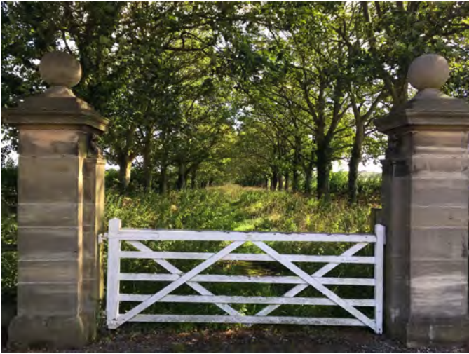
Formal tree-lined avenue leading from Thornton Manor with red sandstone boundary
