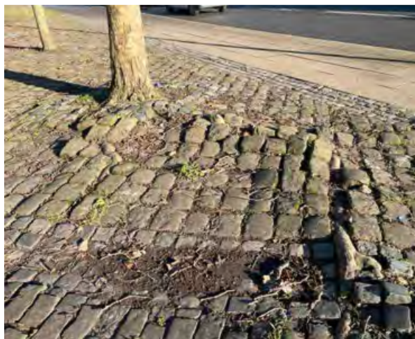
4.3.24 Paving disrupted by concrete blocking
