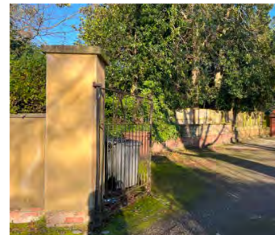
4.3.30 Poor quality rendered pier
