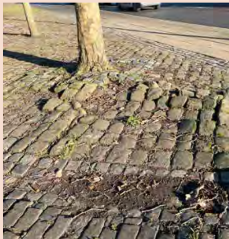
6.2.15 Cracking and damage to paving by roots
