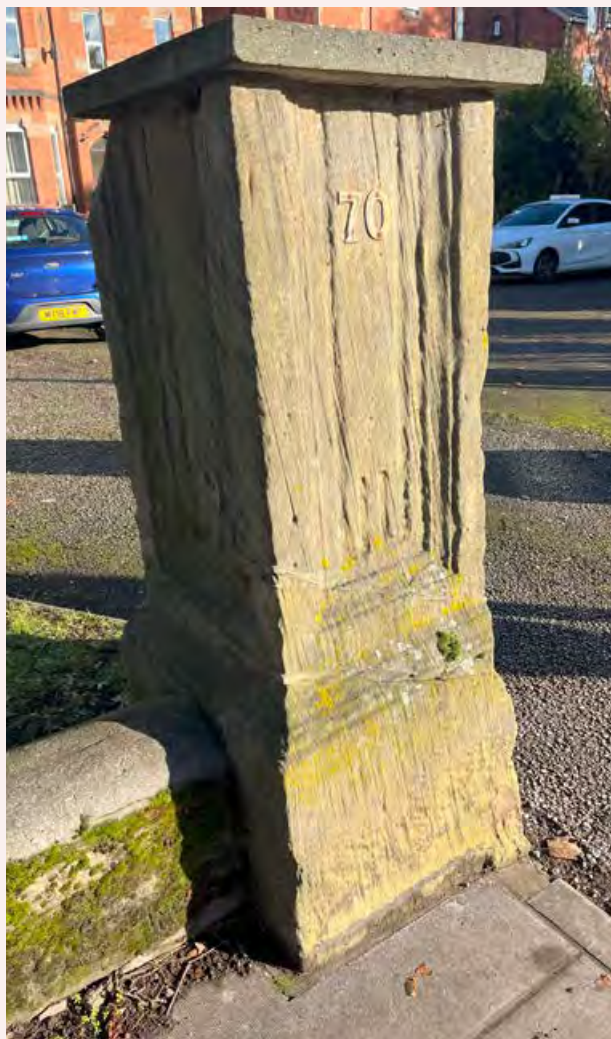
6.2.12 Damage to historic gate pier
