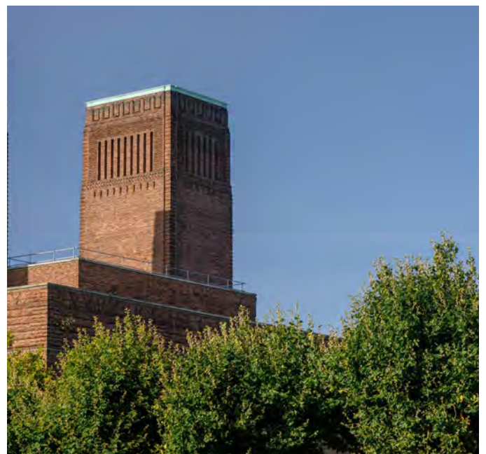
Ventilation Tower, Sidney Street, Birkenhead
