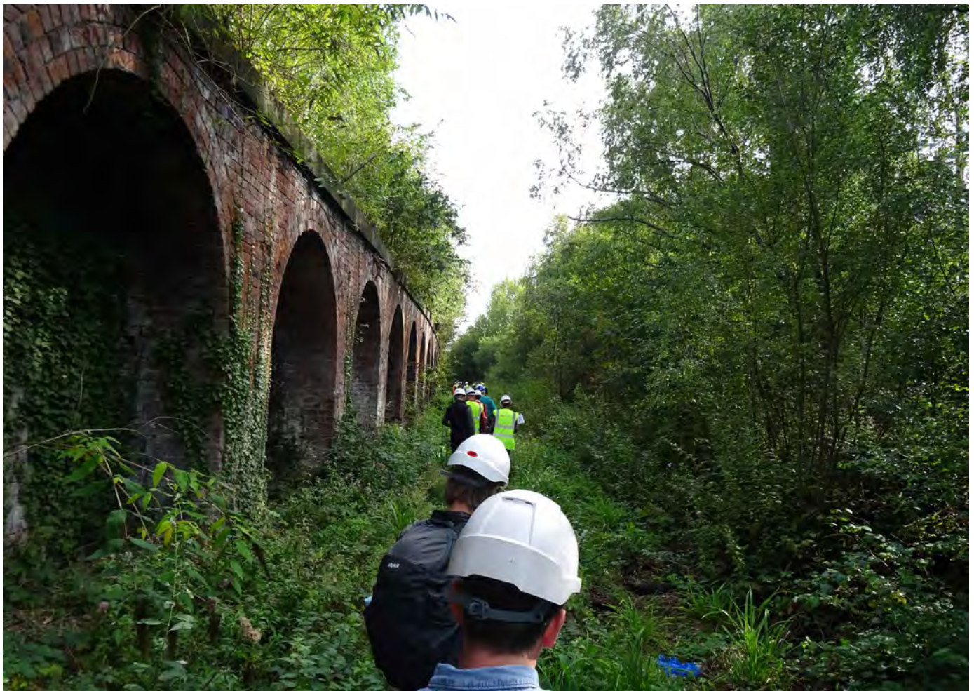
Dock Branch cutting
