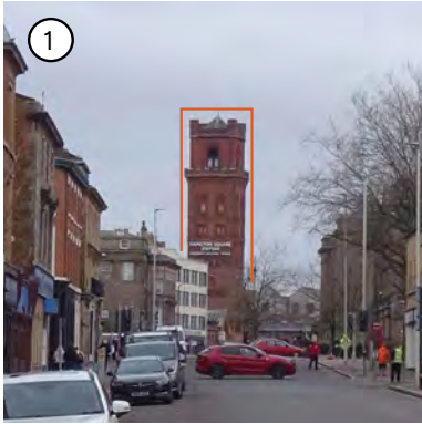
View north towards Hamilton Station Hydraulic Tower from Hamilton Street
