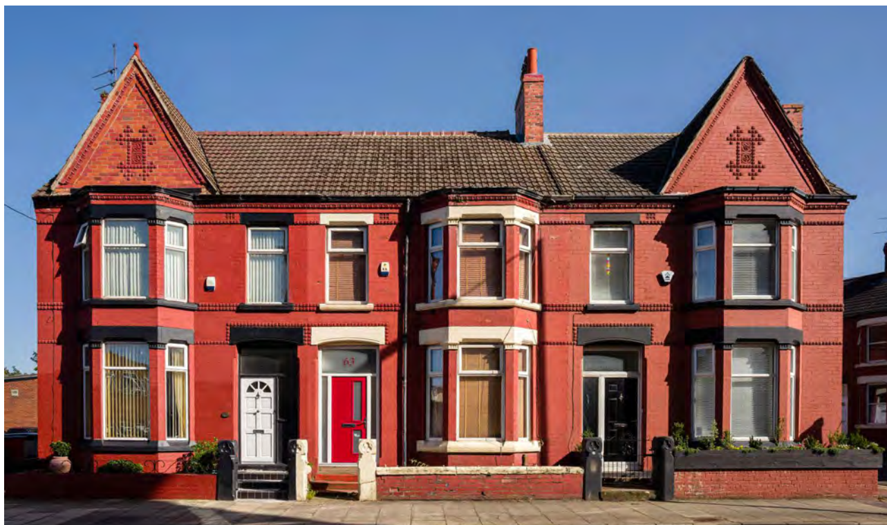
A short run of urban terraces with front gables and fine detailing – an example of Birkenhead's humble, 'everyday heritage'. Photo credit: © PeteCarr
