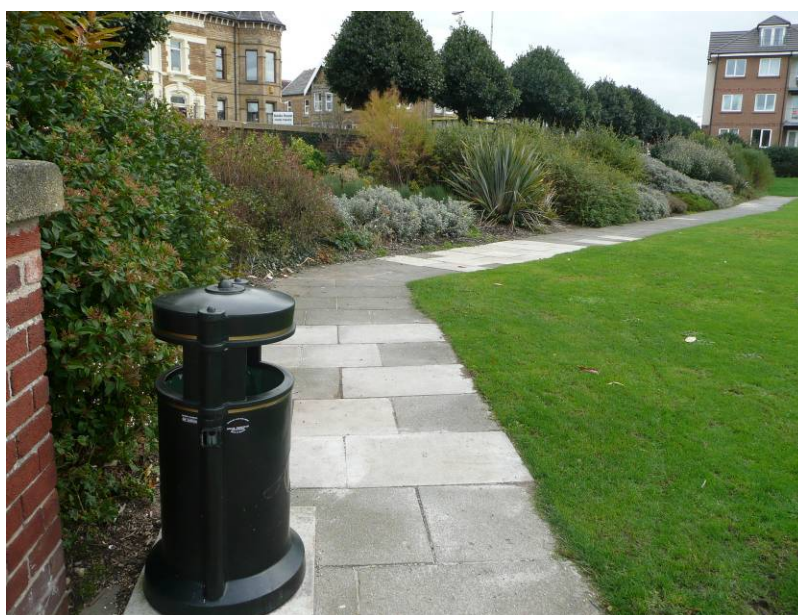
Repaired flagstone footpaths
