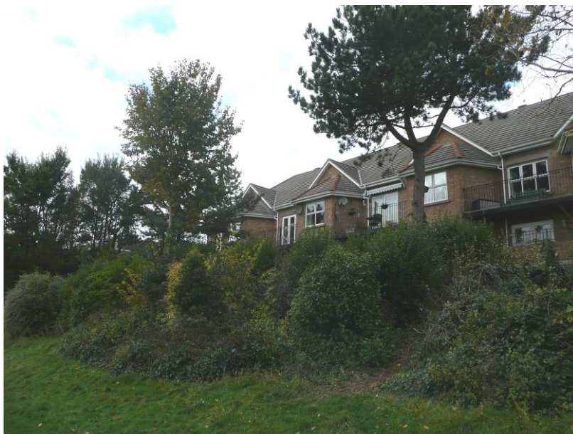
Informal area to northern boundary
