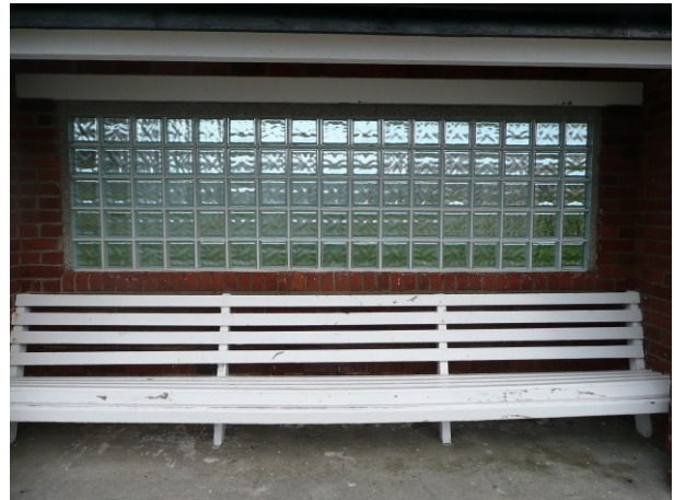
Glass walling block replacement begun in 2011
