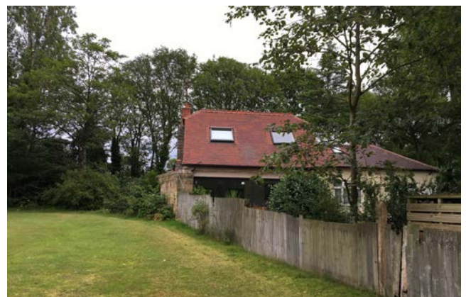
Detached house near the southern boundary of the site
