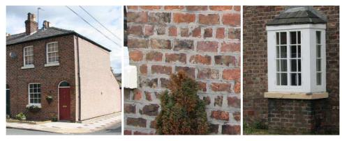
Unsympathetic alterations within the conservation area: (left) pebbledashed end walls to the terraces; (middle) poor quality pointing; (right) the effect of installing double glazing – making the window frames wider, therefore leading to an odd configuration of glazing bars.
