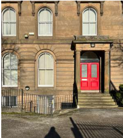
4.3.13 Classical porch with stepped access
