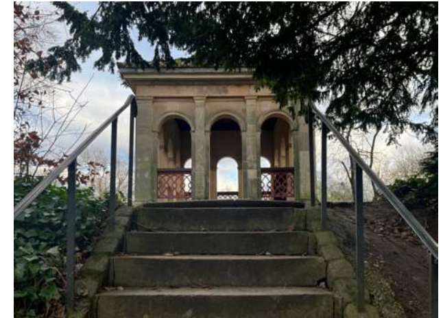
1.6 'Roman Bathhouse' in state of good repair
