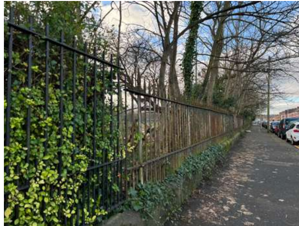
4.12.32 Railings along the road and RUFC
