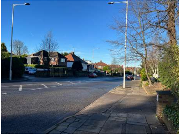
5.1.2 Park Road West semi-detached housing
