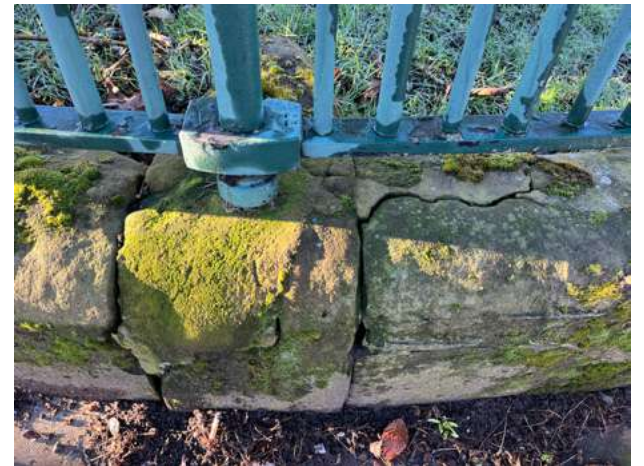
4.3.34 Concrete on stone plinth
