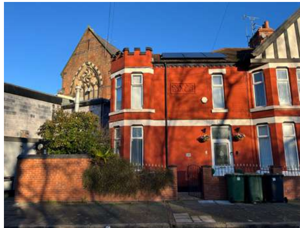
5.1.15 Unusual architectural detailing
