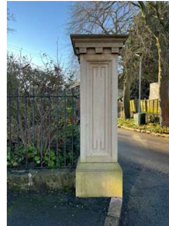
4.3.29 Modern replica stone pier
