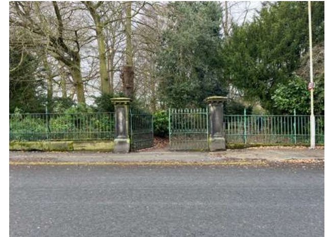
4.6.3 Ashville Road pedestrian entrance
