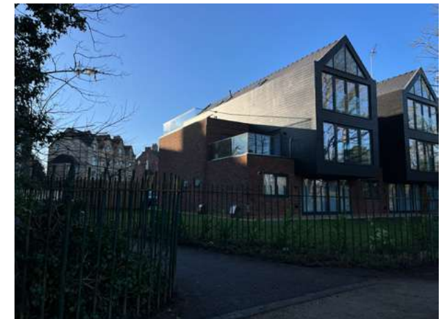
4.10.3 Pedestrian entrance from Park Road South
