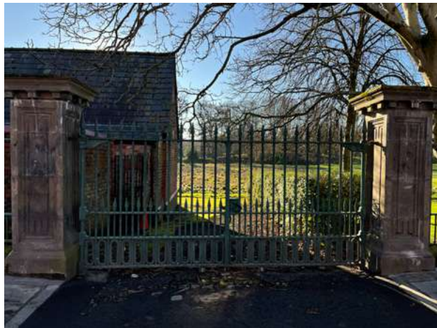
4.12.42 Historic gateposts to Bowling Green
