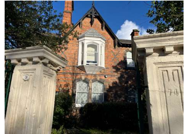
4.12.53 74 Park Road West
