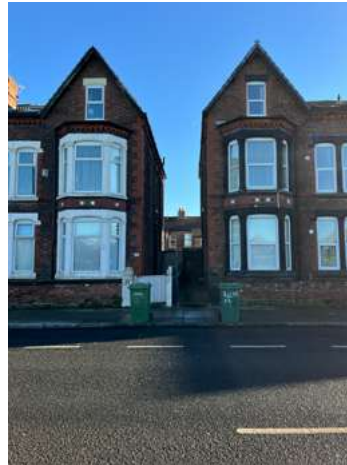
5.1.6 Park Road East with view into back-to-backs
