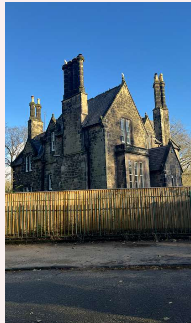
6.2.13 Poor quality modern fencing to boundary
