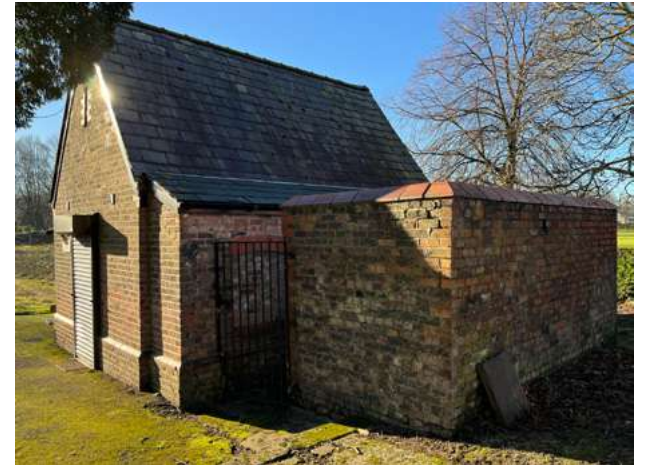
4.11.9 Bowling Green shelter building with shuttering
