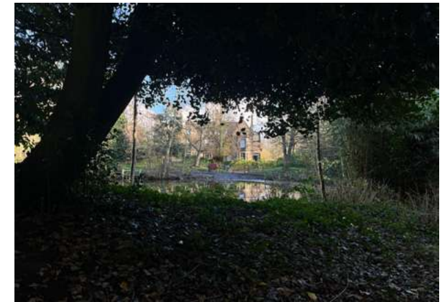
4.1.3 Cavendish Road rear elevations from Upper Lake
