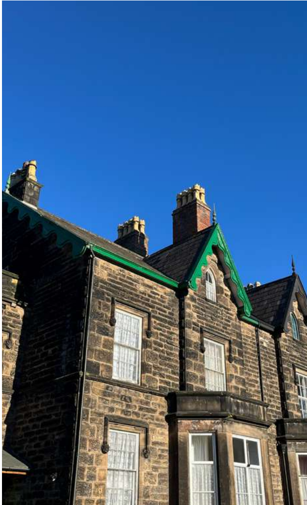
4.3.17 Unusual waved bargeboards and slate roofing.
