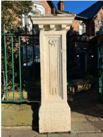
4.3.28 Original stone piers
