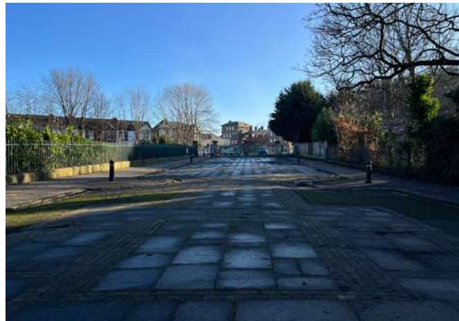
4.3.22 Concrete paving around park
