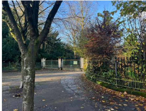
4.6.2 Ashville Road entrance to carriage drive
