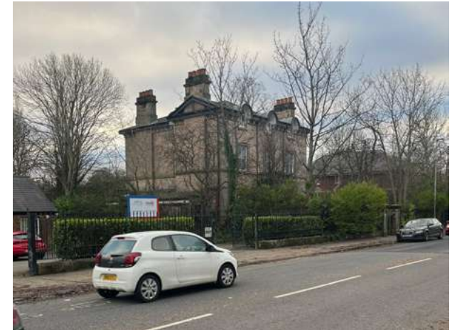
4.12.19 Former Vicarage on Ashville Road
