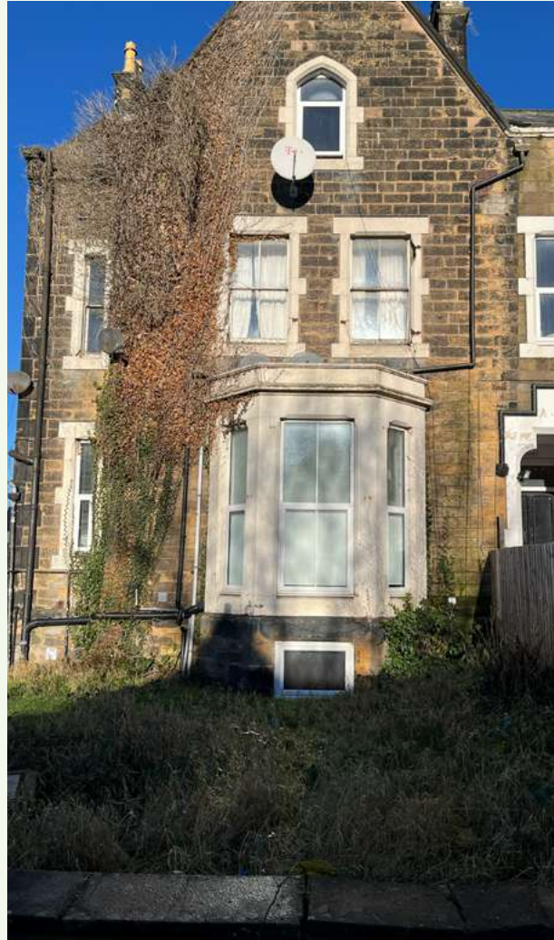
6.2.5 End of terrace showing addition of clutter to facade and loss of detailing
