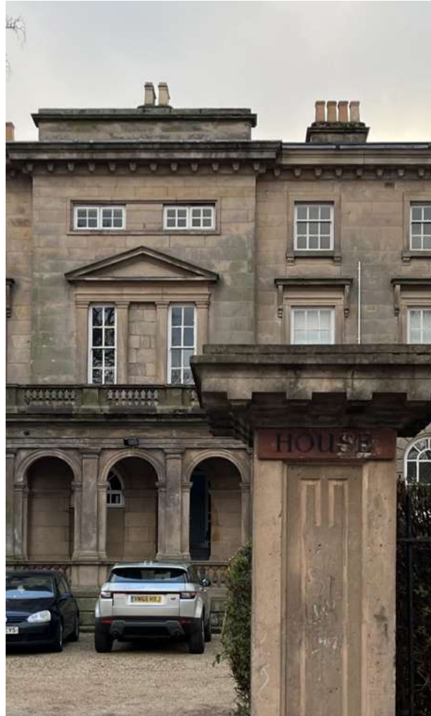
4.3.19 Classical eaves and roof apex obscured by parapet
