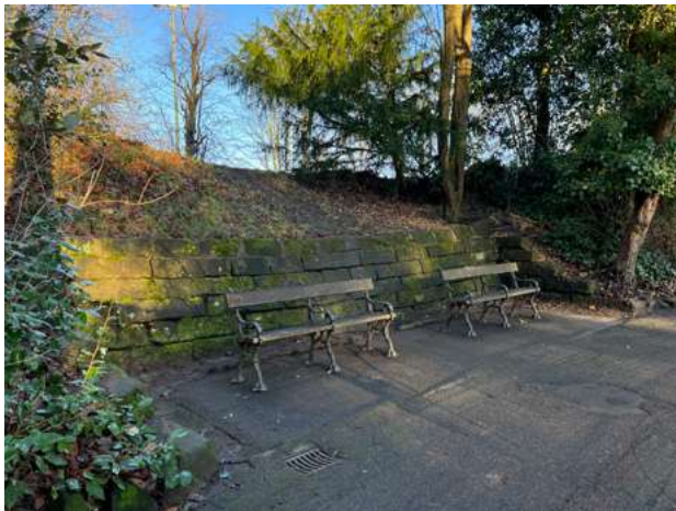
4.6.9 Benches within sandstone niche
