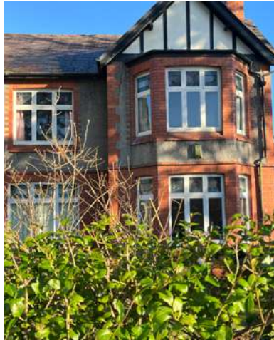
4.3.10 20 th century casement windows
