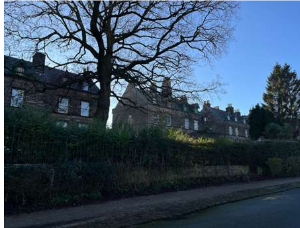
4.10.14 View of Park Road South villas
