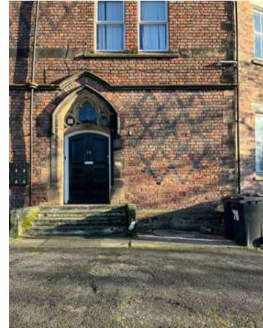
4.3.12 Windowed top light above gothic entrance
