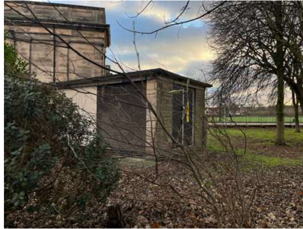
4.12.46 Electrical substation located close to Grand Entrance
