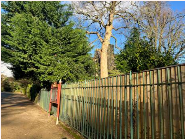
6.2.10 Close board fencing disrupting historic park boundary
