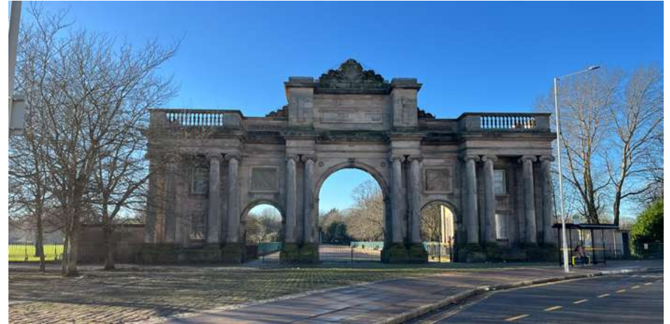
5.2.9 Grand entrance gateway to northeast
