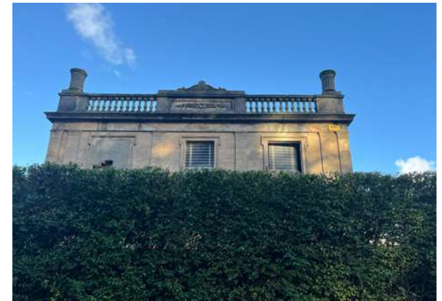
4.3.20 Classical balustrading and parapet
