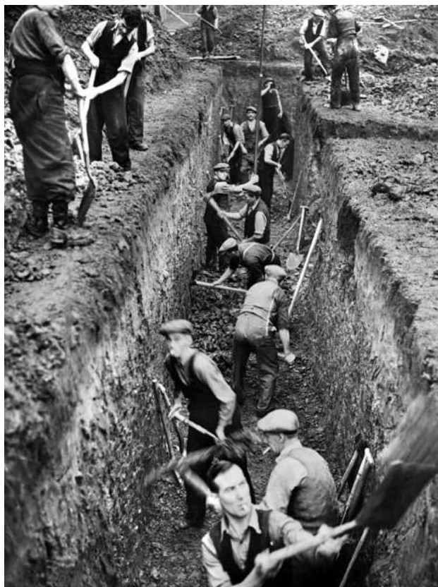
3.12 Men digging trenches, c.1938 ( Liverpool Echo )
