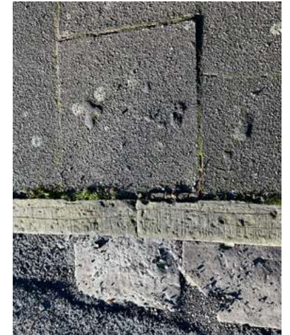
4.3.27 Retained stone edge to paving
