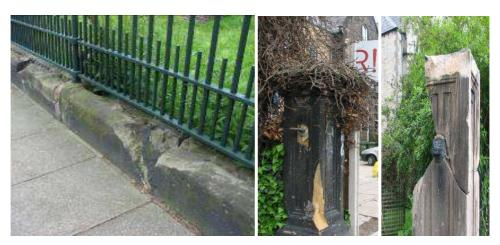
(Left) Damage to original stone plinth; (Middle) dirty / damaged original gatepost that could be carefully repaired; (Right) although a large section of this gatepost has been lost, the remainder is in a fair condition and should be repaired by carefully drilling out any rusting ferrous fixings and piecing in a new section. This may be cheaper than replacing the whole post in reconstituted stone.
