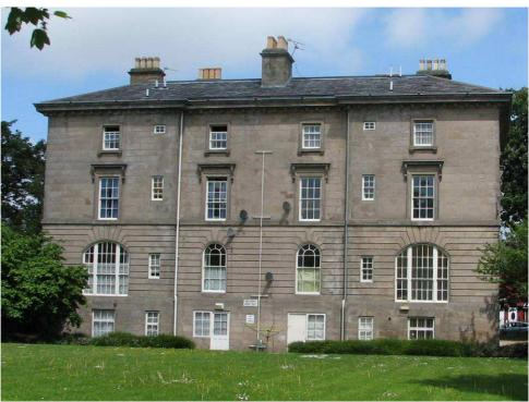
The effects of multiple occupancy on the park-facing side of Roden House. There are additional waste pipes, vent pipes through the roof, a number of satellite dishes and signage on the building.
