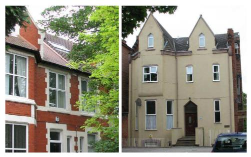
(Left) photograph showing the detrimental effect replacing roof coverings can have on the appearance of a pair of buildings and the awkward detail it results in at the join; (right) a late 19<sup>th</sup> century building that is barely recognisable as such as a result of changes including the installation of UPVC casement windows, the rendering of the front façade and the use as concrete pantiles as a roof covering.
