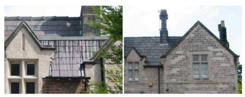
(Left) The photograph shows an example of a particularly poor quality repair that is severely detrimental to the appearance of a listed building. The bitumen used to adhere the felt over the ridge (in itself detrimental to the building) has dripped down over the slate, almost certainly cause irreparable damage. (Right) Excessive and probably unnecessary mortar repairs of the face of the stonework.
