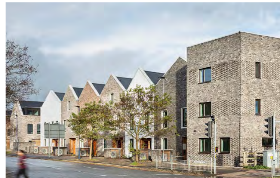
Figure 3.3.2.1 - Marmalade Lane Cohousing Development, Mole Architects
