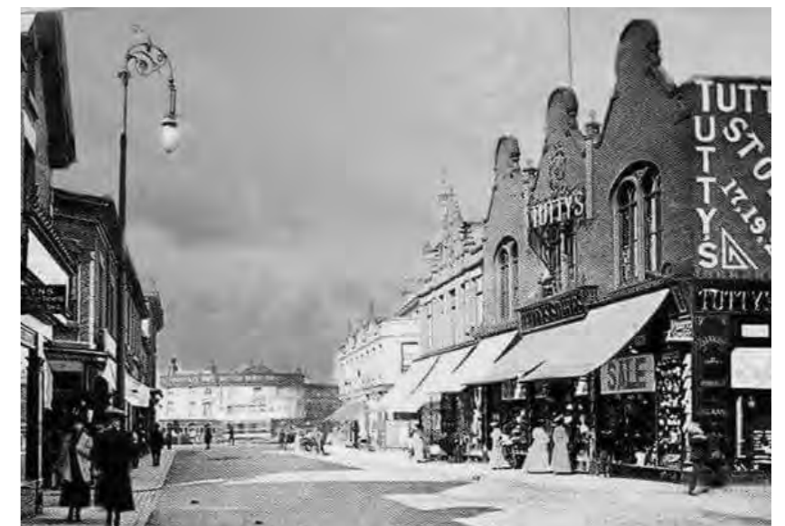
Figure 1.5.15 - Historic view of Oxtan Road looking to Charing Cross
