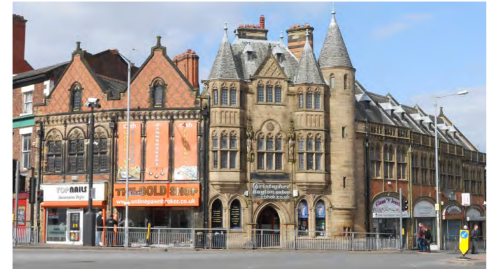
Figure 3.3.7.1 - Bank Buildings, Charing Cross
