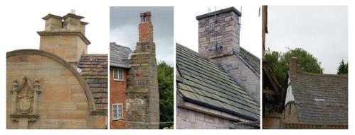
Chimneys in the conservation area; (1) Clover Cottages (2) stone with sections rebuilt in brick seen extensively (3) simple copings to stone chimneys(4) plain brick stack.
