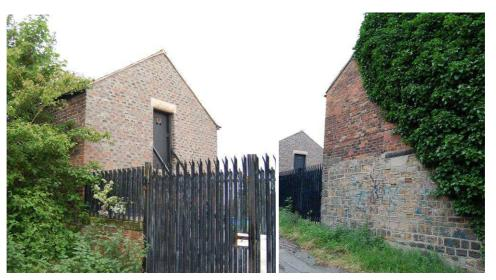
(left and right) poor quality pointing to stone and brickwork as well as highly detrimental palisade fencing at Ivy Farm.
