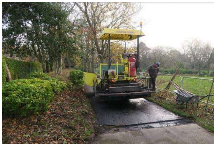
Resurfacing work to upper park 2019
