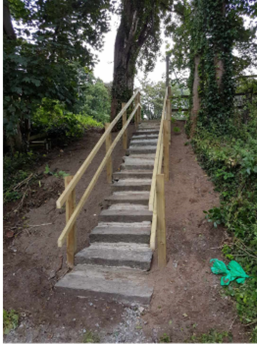
Steps to the upper park were re-bedded in 2021 and a handrail added
