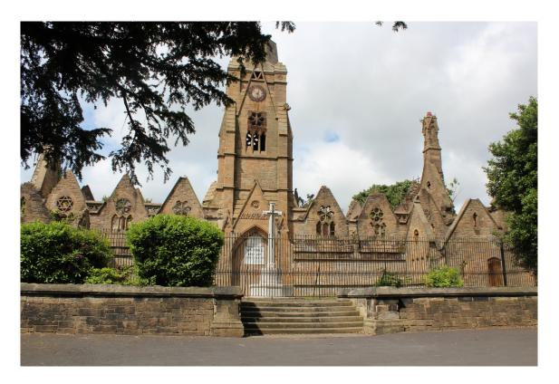
The chapels, one for Anglicans and one for Non-Conformists are joined by a central entrance beneath the originally imposing spire. Each had a nave, aisle, side chapel, outer porch and apsidal east end. The spire was partially taken down and the roof removed in 1980s and the chapels are in very poor structural condition. However, recent works to consolidate the building fabric have revealed that many internal features, including carved stonework and decorated tiles do survive.
