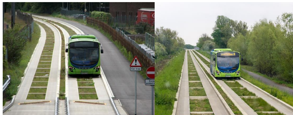
Figure 8: Cambridgeshire Guided Busway
