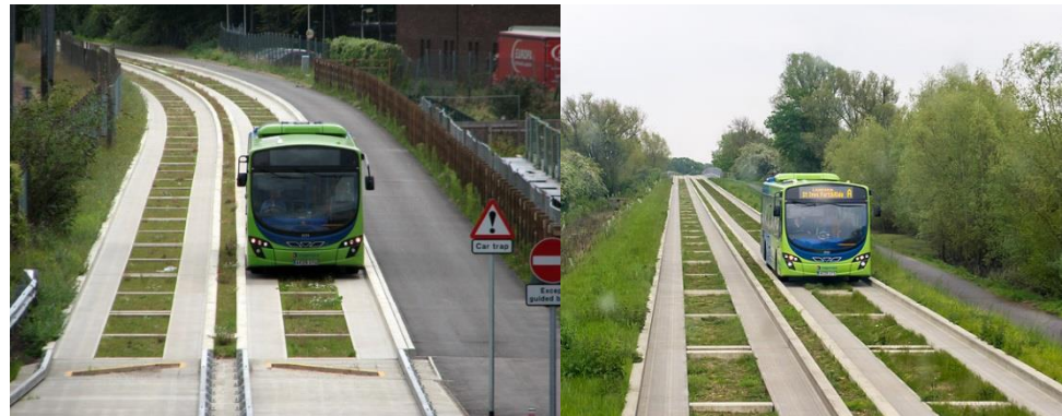
Figure 11: Cambridgeshire Guided Busway
