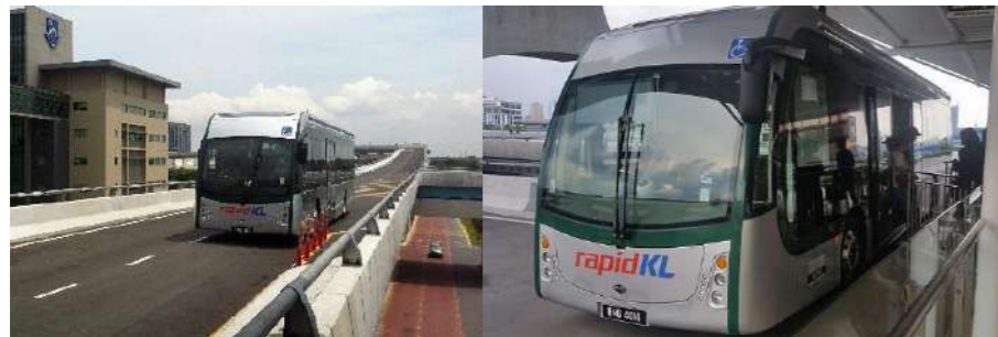
Figure 11: BRT – Sunway Line
