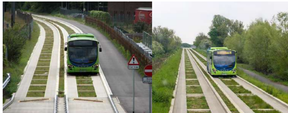
Figure 11: Cambridgeshire Guided Busway
