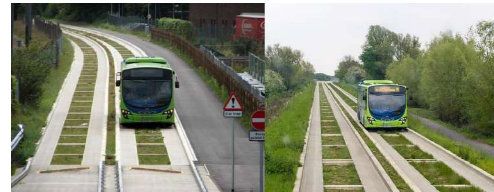
Figure 13: Cambridgeshire Guided Busway
