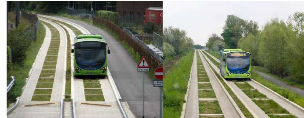
Figure 13: Cambridgeshire Guided Busway
