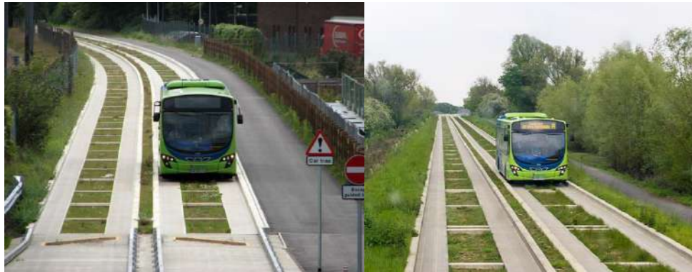
Figure 11: Cambridgeshire Guided Busway
