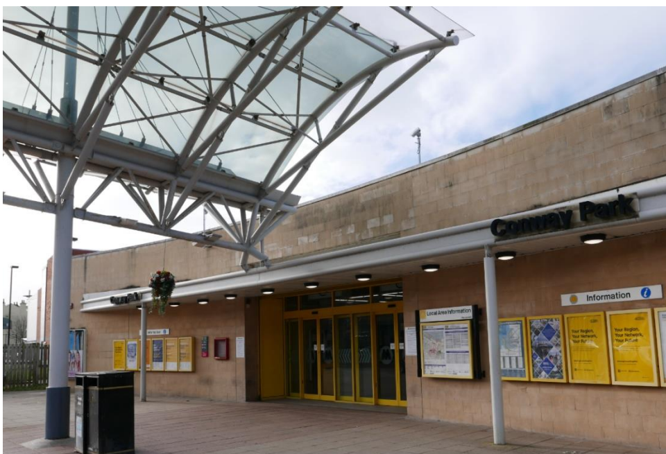
Photo 6: Conway Park Rail Station
