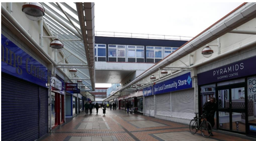
Photo 1: Buildings of low grade within Birkenhead Town Centre
