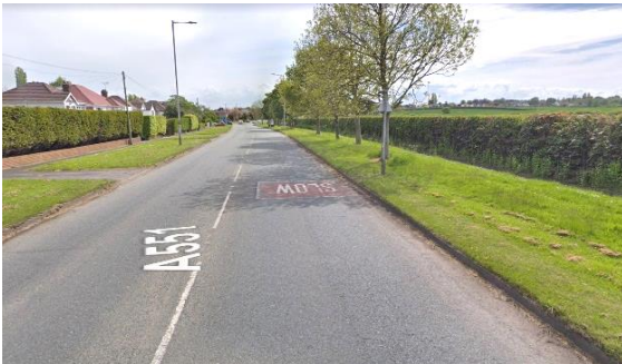
Figure 3.1: A551 Barnston Road
