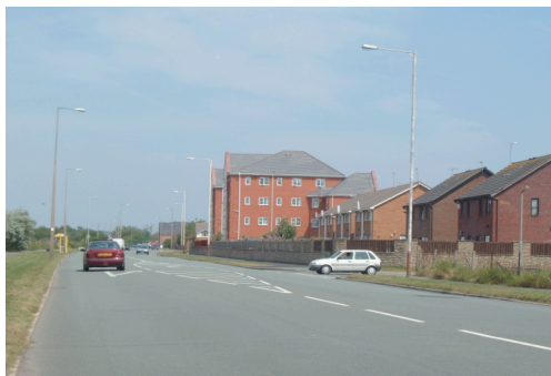
Unacceptable transition between scale and height of buildings
