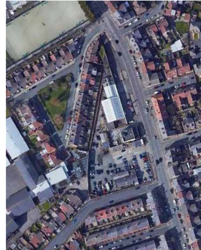
Existing site condition
