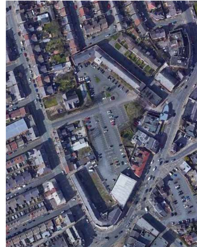
Existing site condition
