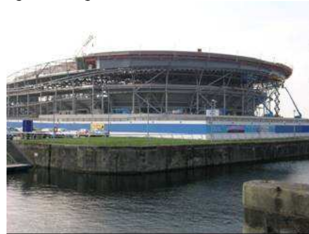
Figure 8.3 Kings Dock Arena
