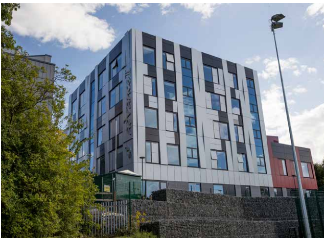
Figure 4.6 - Dudley College's Centre for Advanced Building Technologies (Advanced II)
