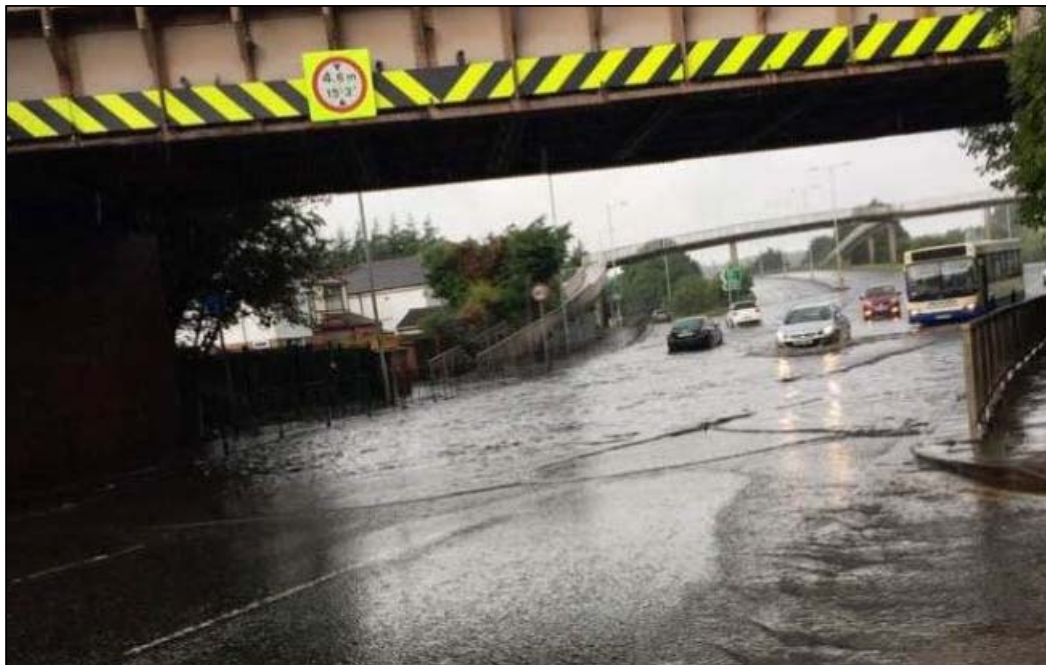
Figure 7: Flooding at Woodchurch Road, Prenton, 23 rd July 2017
