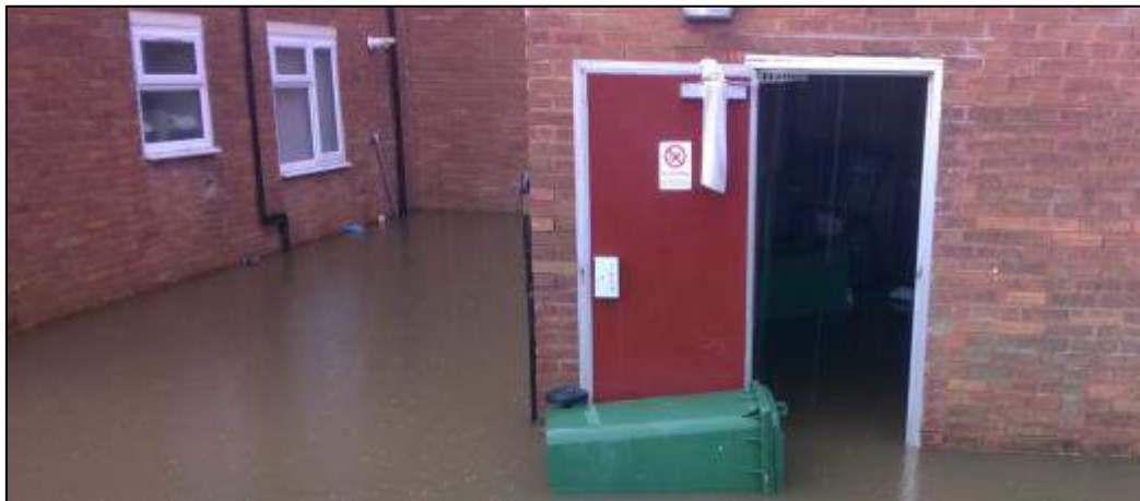
Photograph 5-21 Flooding at Tern Way (2/9/15)
