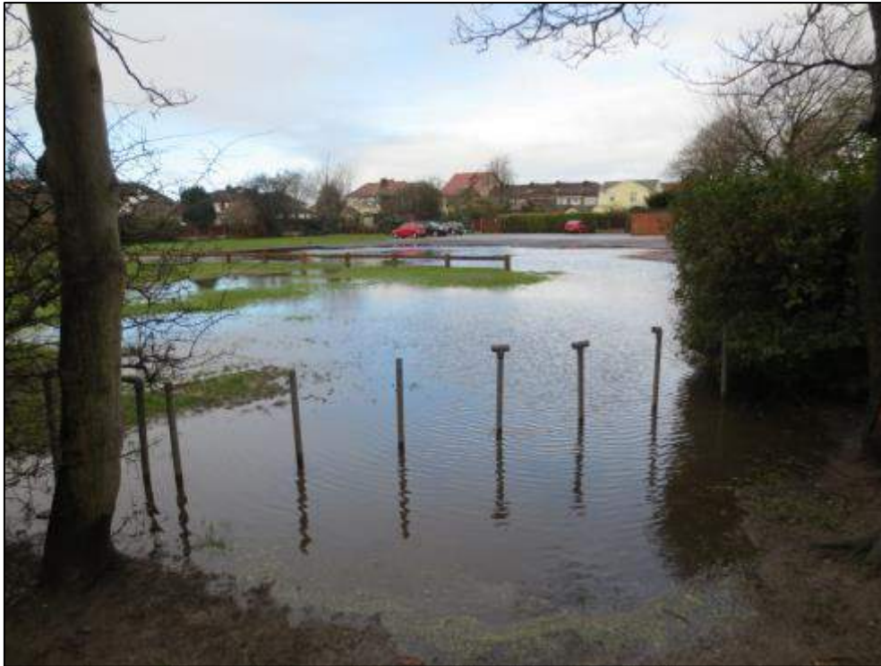
Photograph 5-3 Standing Water in the Coronation Park Car Park (1/3/16)
