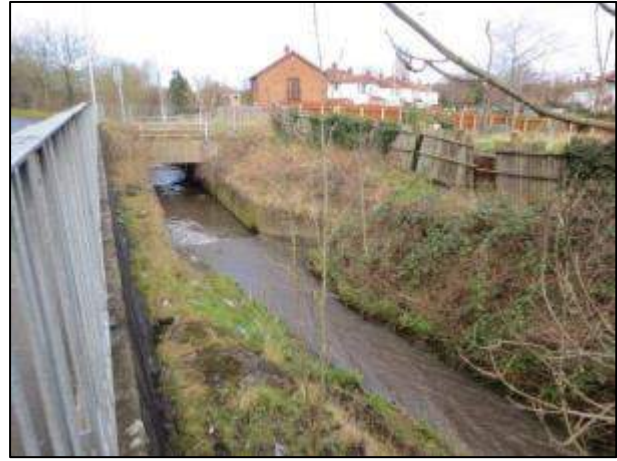
Photograph 5-31 Access Bridge to Durley Drive
