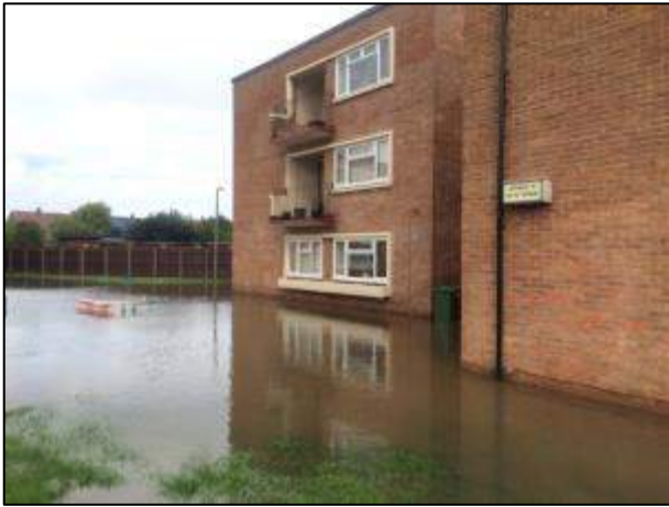
Photograph 5-18 Tern Way Flats (2/9/15)
