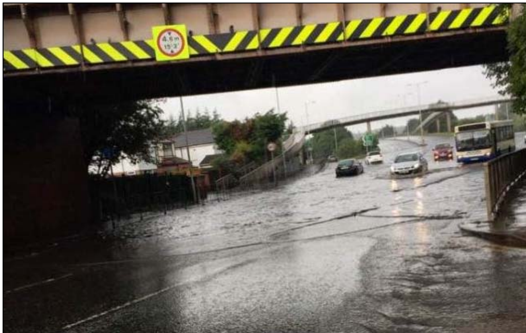
Figure 7: Flooding at Woodchurch Road, Prenton, 23 rd July 2017
