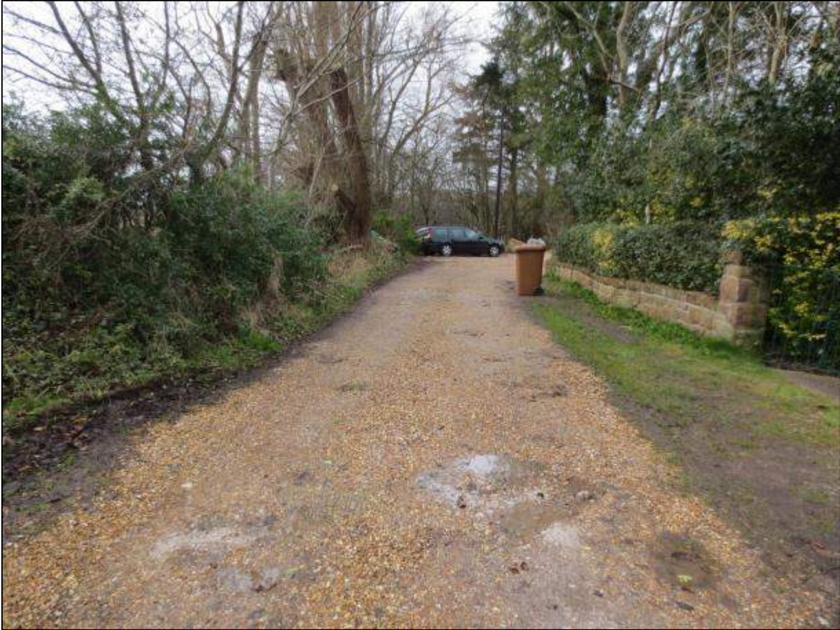
Photograph 5-34 Unadopted Highway on Mayew Road (2/3/16)
