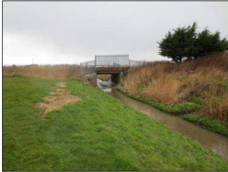
Photograph 5-25 Arrowe Brook Railway Bridge (2/3/16)
