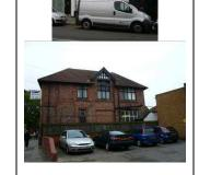
East elevation: Former gable end fronting street, now much altered. Replacement roof of interlocking profiled tiles. Roof now hipped, with loss of projecting gables to east and west elevations.
